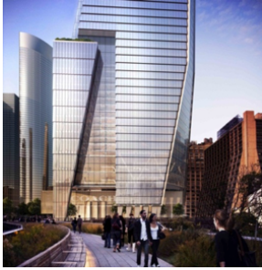
Hudson Yards, LEED Gold South Tower
